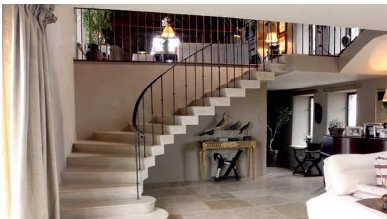
A slimline metal balustrade gives this flight by Ian Knapp Stonemason an open feel. The treads were hand-carved in an off white French limestone, called Roche Marron
